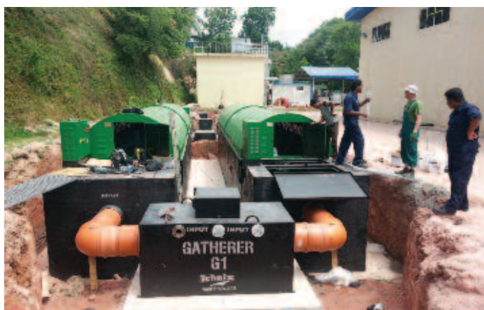
Ugradnja Biorotora kontejnerskog na Sri Lanci Construction of biorotor container type on Sri Lanka
