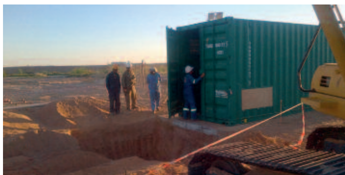
Montaža kontejnerskog Biorotora u Radničkom kampu u Iraku / Installation of biorotor container type in workers camp in Iraq
