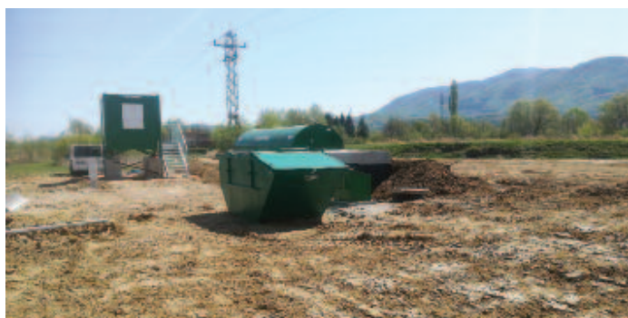
Biorotor, kontejner za prihvat mulja i upravljački objekt / Biorotor, sludge receiving container and management facility
