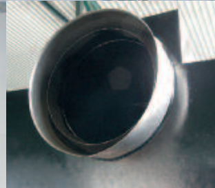
ULAZNA CIEV SEPARATORA SEPARATOR INLET PIPE
