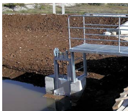
On-site lifting of special separator with lifter
