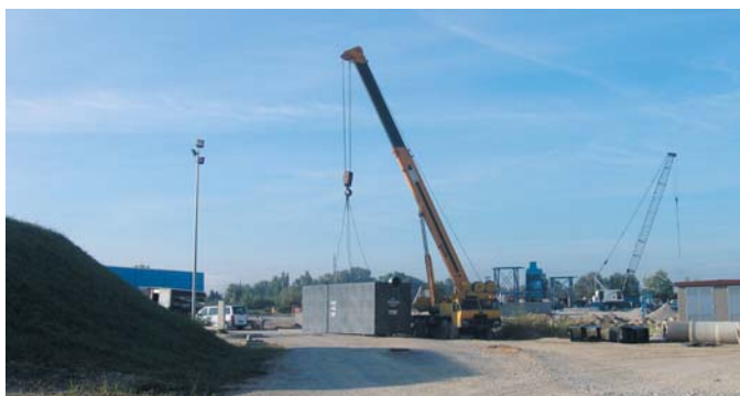
Unloading and installation of Tehnix separator
