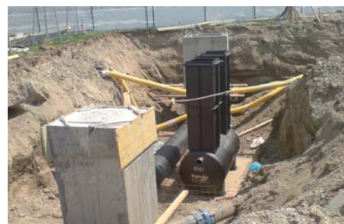
Installation of the special separator
