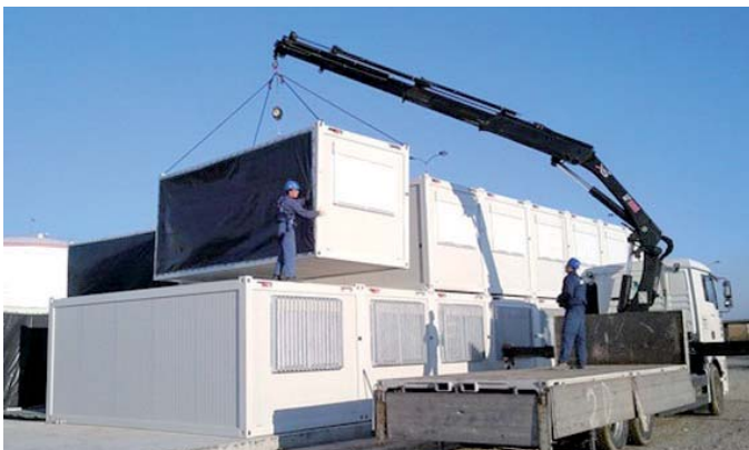
Assembly container settlement on site
