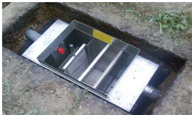
Installation of the grease-trap
